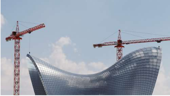
Fig. 17. Rapid assembly of architectural structure. Our geometric approximation could provide the frames around the glass panels which can be fully manufactured off-site, transported flat, and deployed onsite using only two cranes. While our design method is scalable, realizing full architectural deployment requires future engineering studies.
